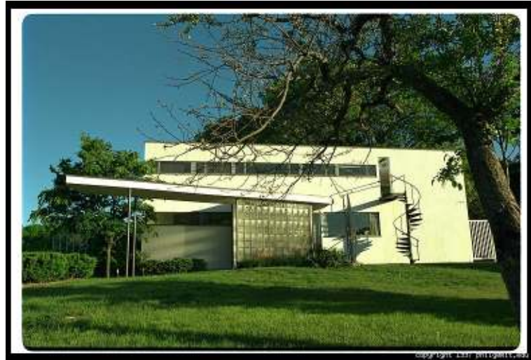
Fig. 3 - 1938 Gropius House, home of architect, Lincoln, Mass.
